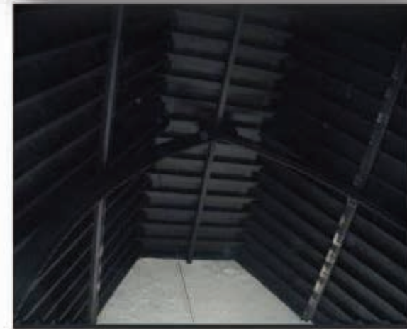
Figure 1 – inside view of existing roof
