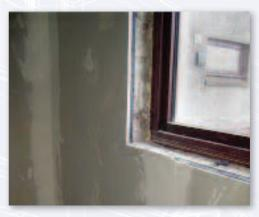
Panels of Spaceloft® 9251 laminated to building facing board were easily attached to apartment walls and around windows and other fixtures.
